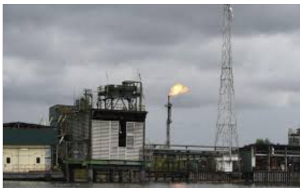
Fig 1: Batan flow station Warri south LGA
