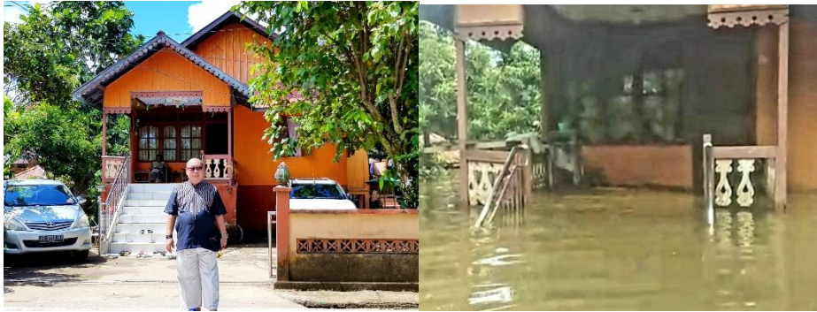
Figure 2: Flood Condition in Sintang, November 2021
