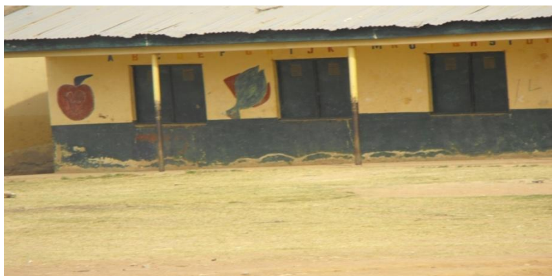
Picture 2: A photo view of the nursery section block of the primary school.
