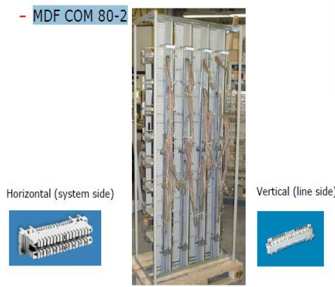
Figure 3 Main Frame Distribution 80-2
