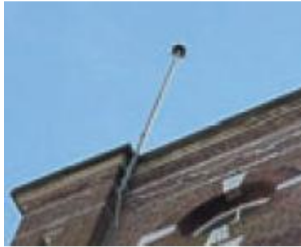
Fig5. lightning conductor with sparkover device.
