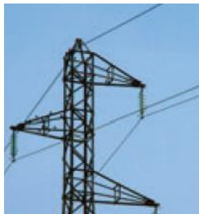
Fig7. Lightning protection by shielding wires
