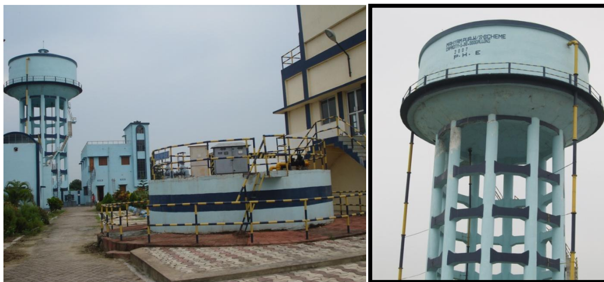
Figure 2.2: Majhyampur Water Treatment Plant
