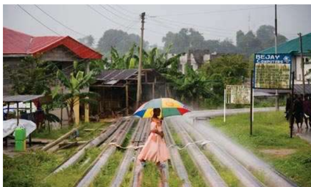
Figure no1: Exposed oil pipelines running through settlements (Uyigüe and Agho 2007)
