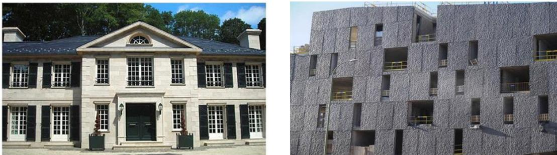
Figure3: (Left) stone exterior cladding (ArchiExpo, 2014); (Right) textured concrete exterior cladding (Architectonic Concrete, S.L., 2011)
