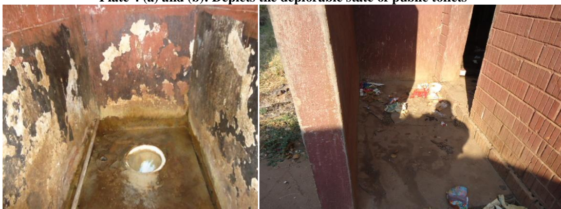
Plate 4 (a) and (b): Depicts the deplorable state of public toilets
