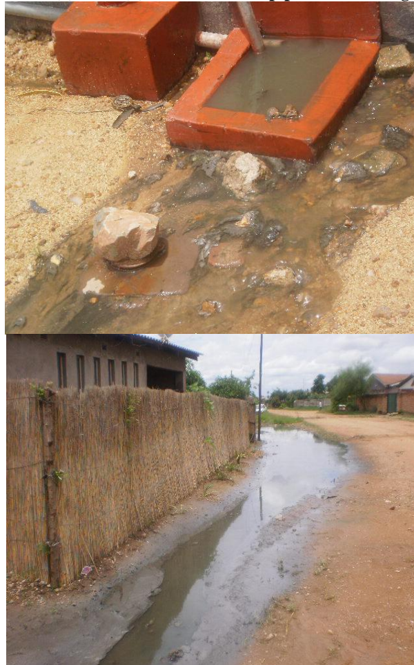
Plate 3(a) and 3(b): Broken sewer pipes and blockages
