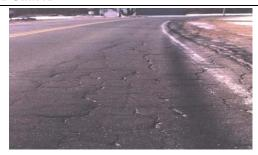
Fig 3. High severity alligator cracking
