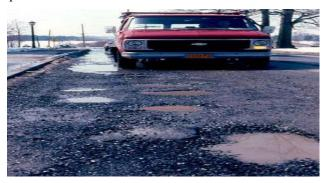
Fig 10. Potholes caused by poor drainage
