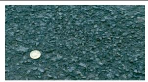
Fig 12. High severity ravelling of asphalt surface
