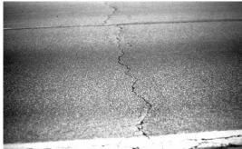
Figure 5. Low severity transverse crack.
