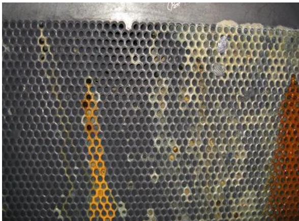
Fig. 1: tube-to-tubesheet failure leads to leakage
