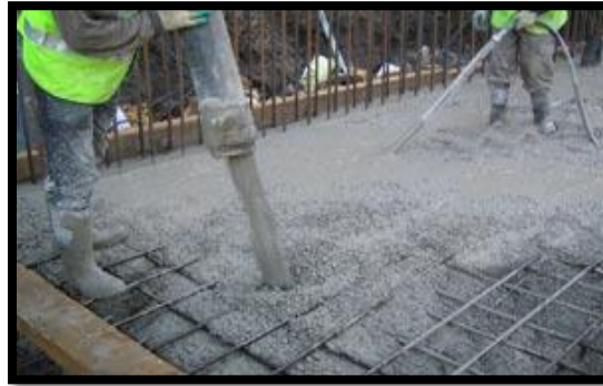
Fig 4: Showing that workability is more and pumping will be easy.
