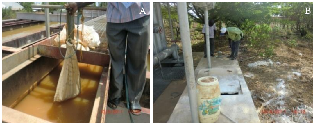
Figure 11: (A). Improper dosing of coagulant (alum) at Ibi-Wukari water treatment plant, (B) Inspecting improper dosing of disinfectants (HTH) at Ibi-Wukari water treatment plant.
