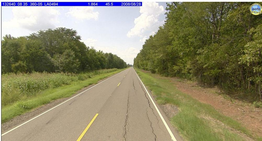
Figure 3: Pavement distresses [Source DOTD]
