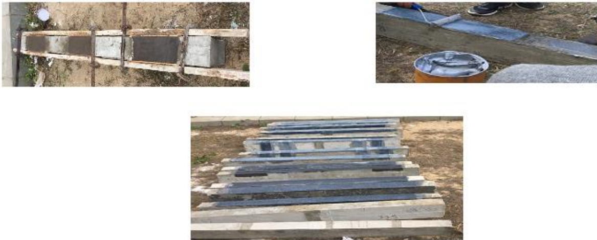
Fig. 5 the application of epoxy to the concrete surface for CFRP sheet bonding.
