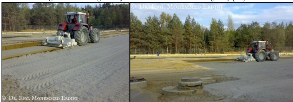
Figure 1: Blending the layer from soil-cement in the highway project
