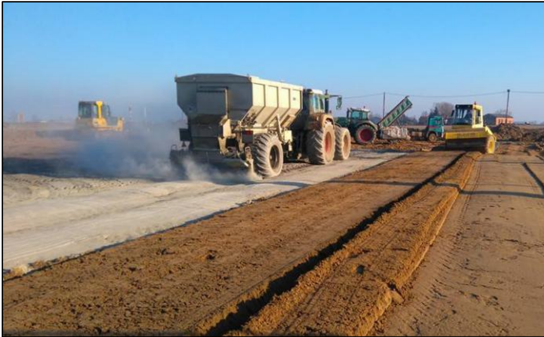
Figure 3: Deployed the layer from residues cement in the highway project
