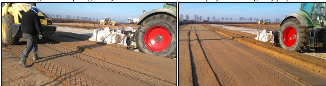
Figure 2: Preparing the layers before residues cement deployed in the highway project
