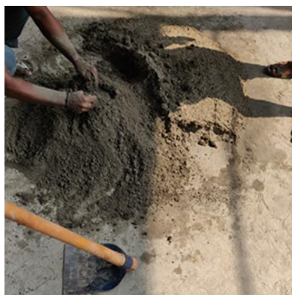
Fig 3: Mixing cement, sand and water
