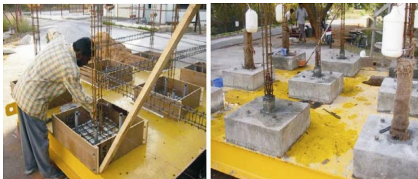
Figure4.1 (a) & (b): Casting of Footings
