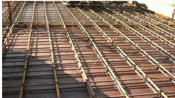
Figure 4.3: Slab reinforcement
