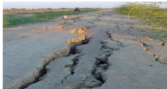
Fig. 12: Cracking and inelastic deformations of crest of the embankment dam caused by the 2001 Bhuj earthquake in India. The prediction of cracks and damage requires nonlinear dynamic analyses and modelling of dam materials. It was sorted by [18].
