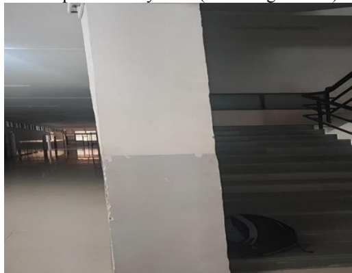
Fig.No.4.5 Undamaged Column.
