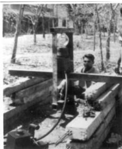
Fig. 7. Experimental set-up for in-situ pull-out capacity
