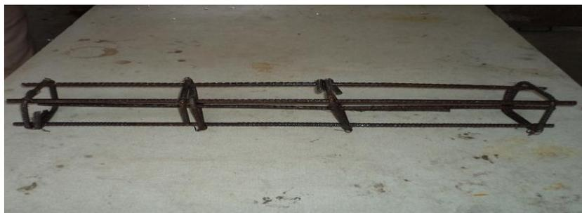
Figure-II Conventional RTS Bar fabrication
