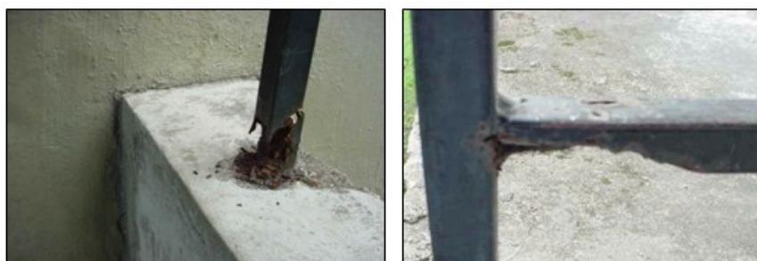
Figures 13, 14 – Appearance of atmospheric corrosion of carbon steel rods.
