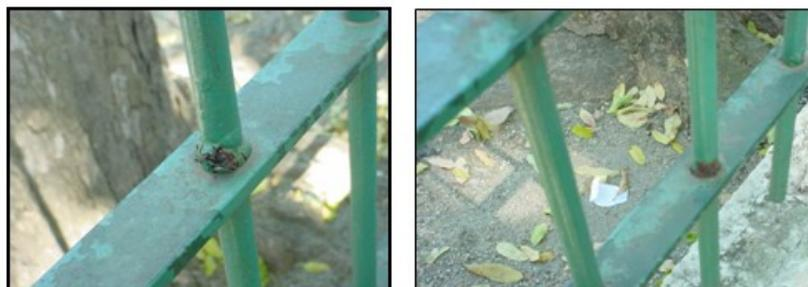
Figures 7, 8 - Aspect in grating corrosion of carbon steel coated with green paint.
