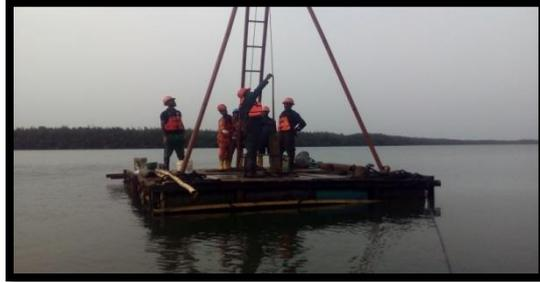
Figure 2: Over water Geotechnical Investigation for Sand at Kalaibama Creek
