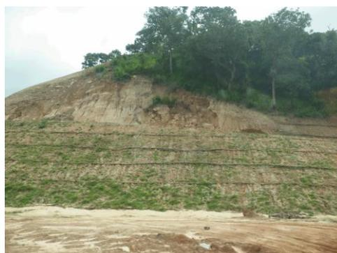
**Figure 3:** A slope near Nsukka Southeast Nigeria revealing failure on a remediated portion (photo by Fukuoka)
