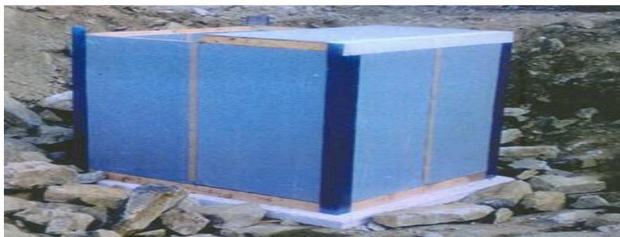
Figure 2. The completed seismic vault platform anchored to the bedrock.
