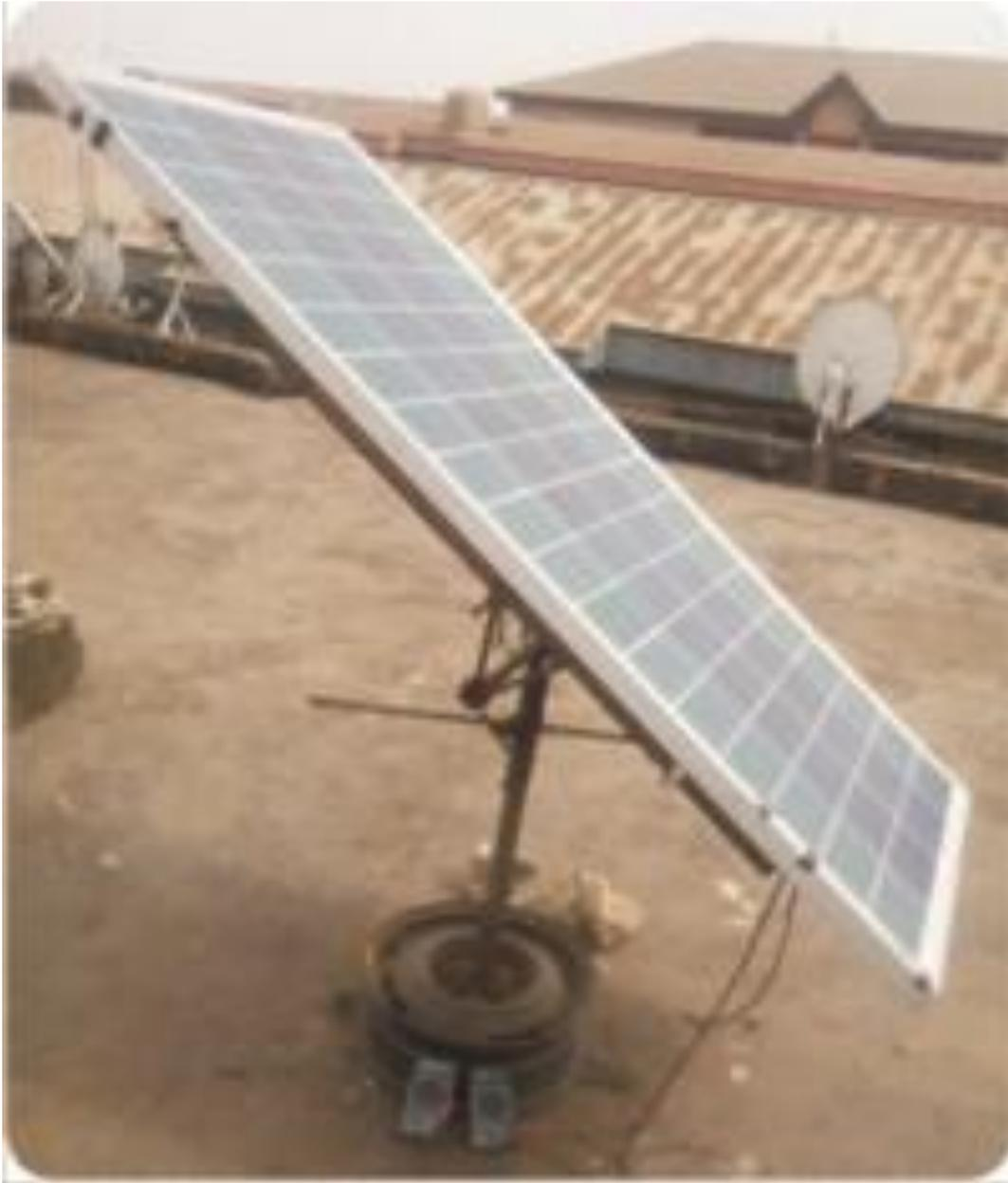
**Fig..4 Picture of the Tracking mounted Panel**
