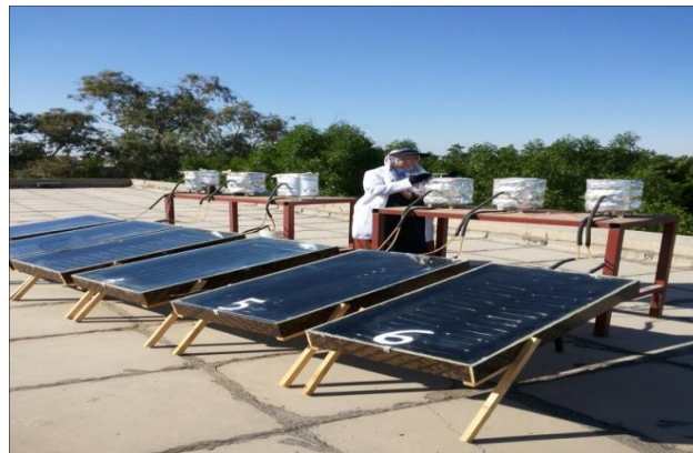
Figure (3) A photograph describes the work of the solar collectors .
