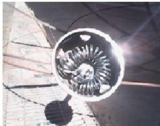
Figure 5: Coiled copper tube inside the absorber
