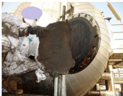
**A bulk of scale extracted during Routine maintenance**
