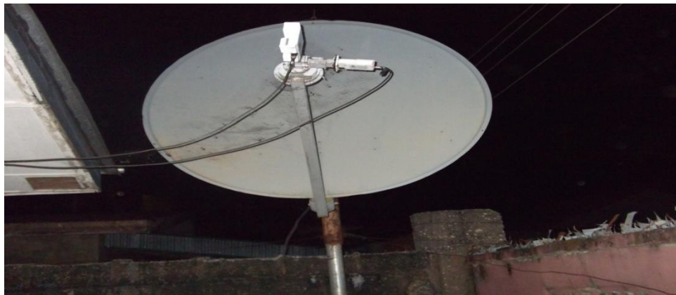
FIG 1-TELECOMMUNICATIONS INFRASTRUCTURES SUPPORTING ICT
