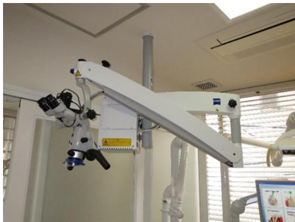
Figure 5: ceiling-mounted supporting structures
