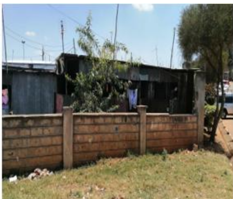
PLATE 8: A section of the short perimeter wall
