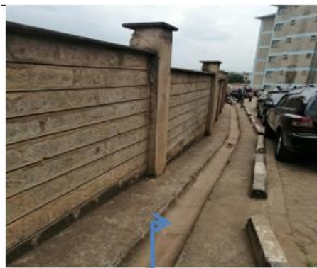
PLATE 11: Storm water drainage subway
