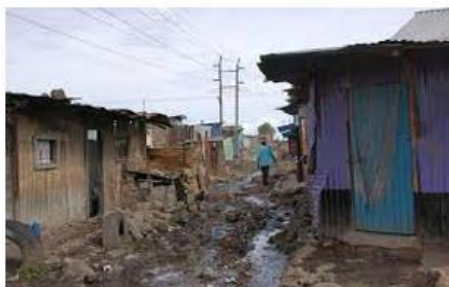
PLATE 1: A section of the road before upgrading
