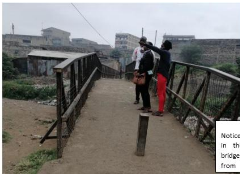
PLATE 4: Constructed foot bridge
