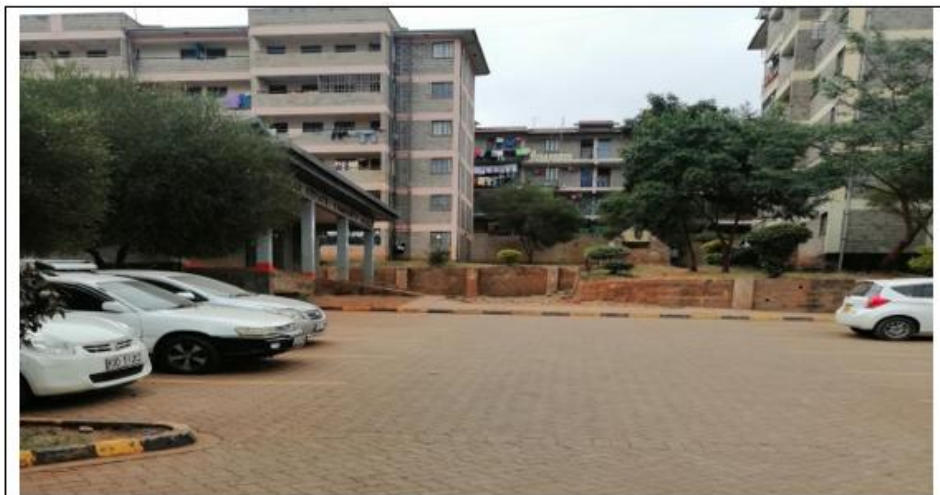
PLATE 10: Paved cabro road
