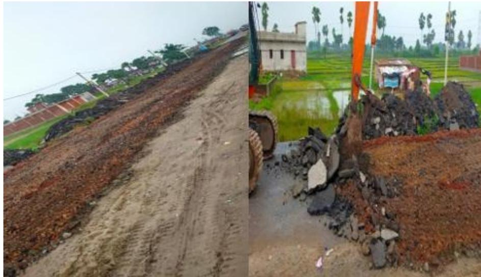
Fig.1.1 Dismantling of DBM Layer of Road Surface
